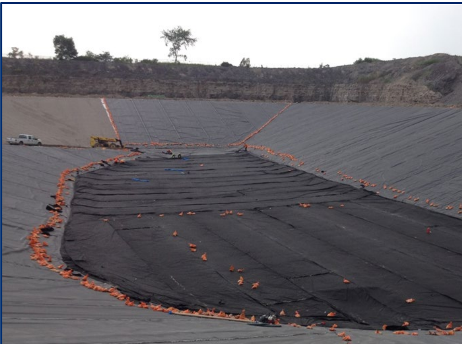
This is a photo of the 2012 engineered landfill cell under construction.
